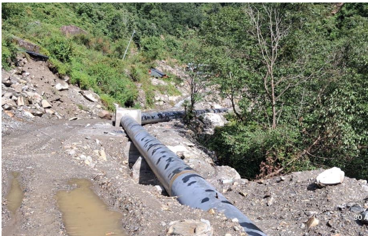
Figure 5: Headworks works progress.
