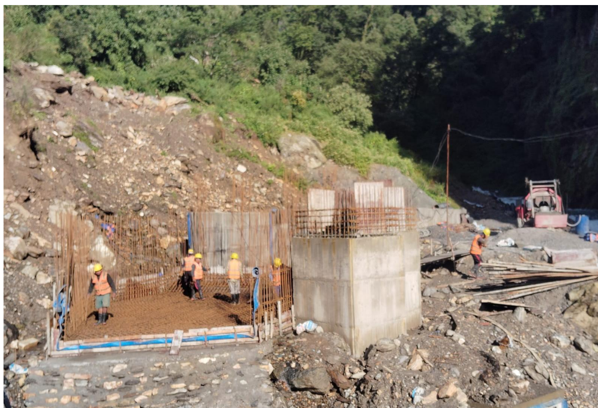
Figure 2: Hedapond Work Progress
