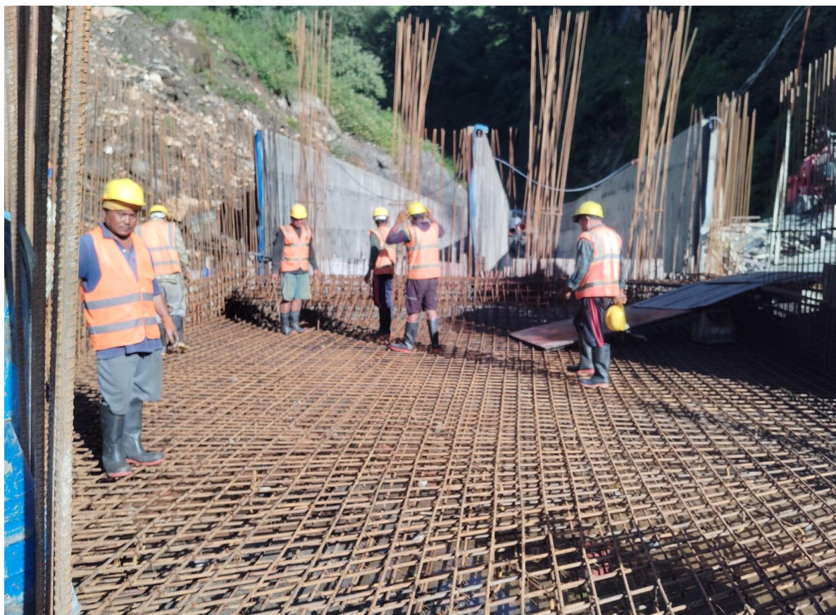
Figure 3: Hedapond Work Progress
