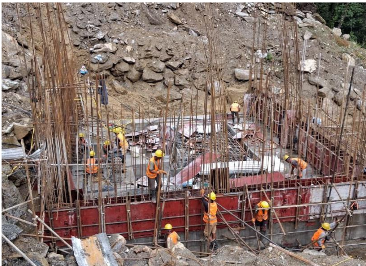
Figure 11: Powerhouse works Progress (Shear wall formworks)
