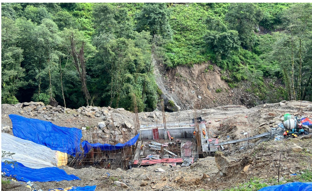
Figure 12: Powerhouse Works Progress (Bay 1&2 machine hall raft)
