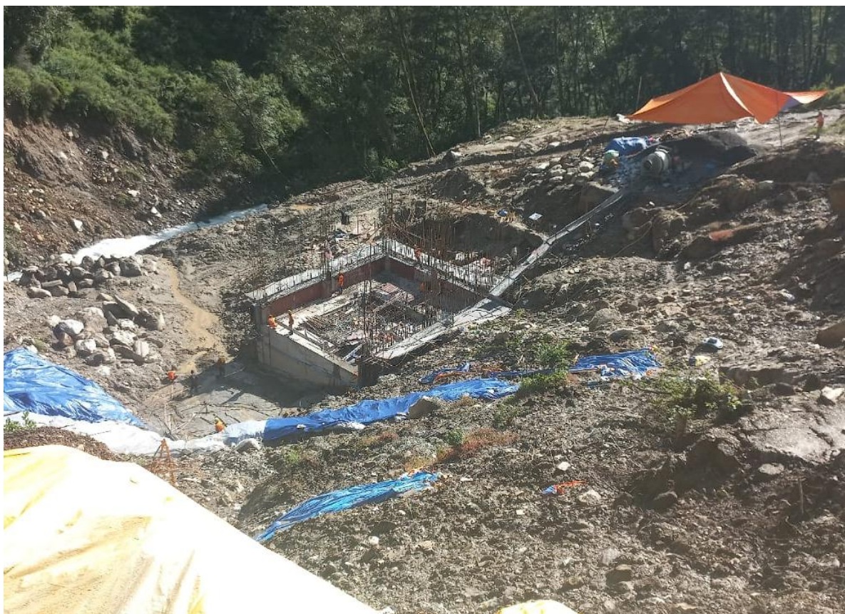
Figure 13: Powerhouse Works Progress.
