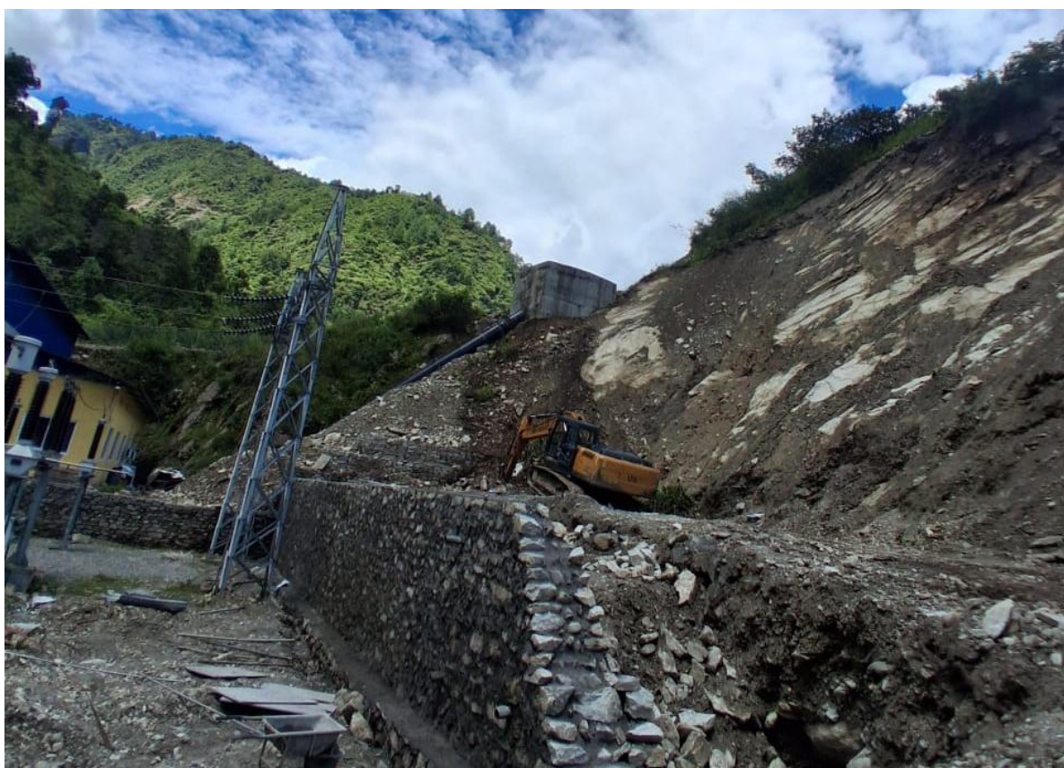
Figure 14: 33/132KVA sub station protection works at shoring khola.
