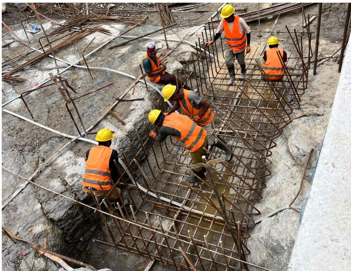
Figure 8: Powerhouse Machine hall rebar works.
