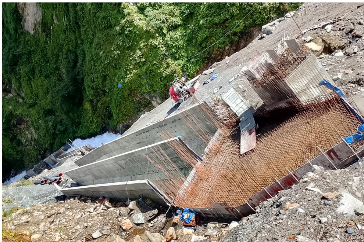
Figure 1: Hedapond Work Progress
