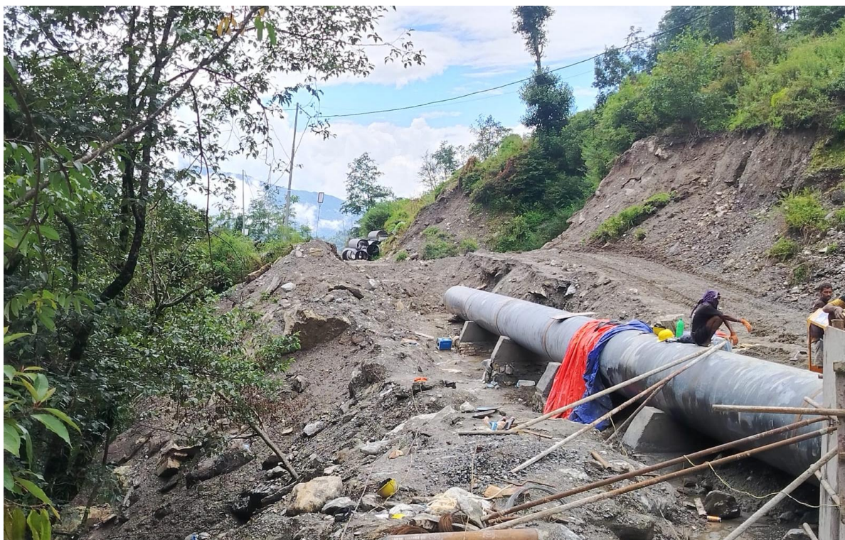
Figure 7: HRP erection is ongoing,
