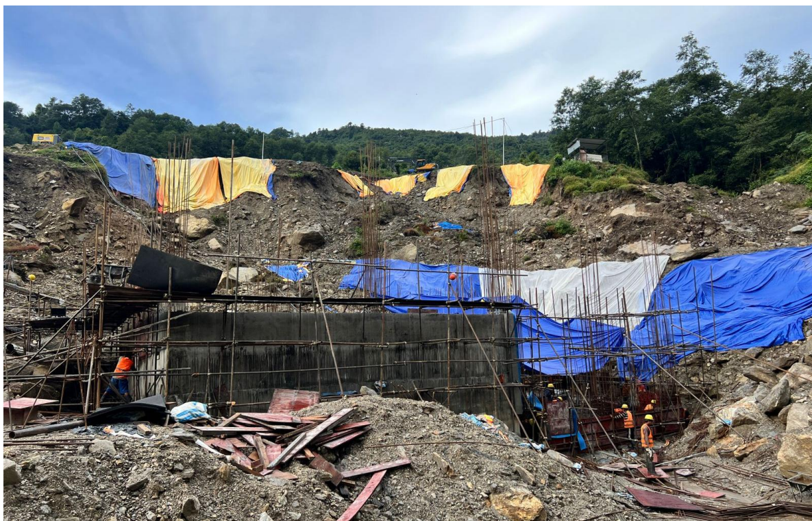
Figure 9 : Power House Work Progress.
